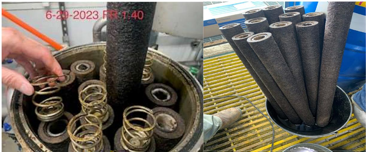
Fig. 10—Cartridge filters (individually new on the right; installed in the housing on the left).
